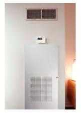
Installs in a small mechanical closet and can be ducted to multiple rooms.
